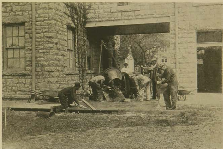
CONCRETE MIXING
