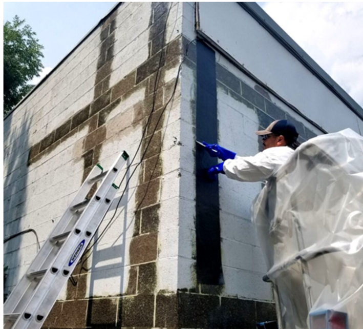
Figure 12: CFRP on Exterior of Masonry Building
