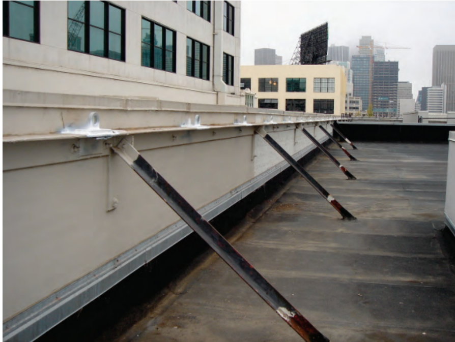
Figure 14: Parapet Bracing
