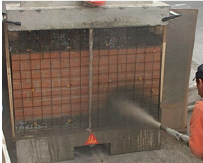
Figure 25: Shotcrete Being Installed
