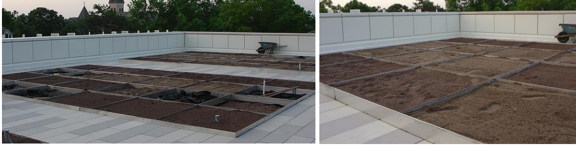
Figure 2.2. Substrate Application on the APD-EGR, with most of the 6-inch and 8-inch Beds Shown. In the photo on the left one can see the filter fabric that is being placed atop the BuildEx Haydite® drainage layer, with the two different substrate mixes then placed atop the BuildEx Haydite® drainage layer, with the two different substrate mixes then placed on top of the fabric separator within each of the 72 green roof plots. Photos by Lee R. Skabelund (July 18, 2017).
