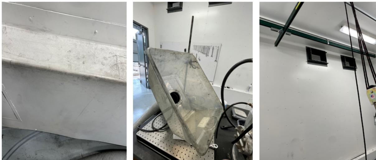
**Figure 2.2:** *On the left, the steel curtain protecting the passthrough for the gas tubes (shown passing under the curtain) and the entrance to the ducts on the east wall is shown. The middle depicts the snorkel device set up adjacent to the reactor vessel, and the right depicts the steel wall and make-up air vents on the west wall.*
