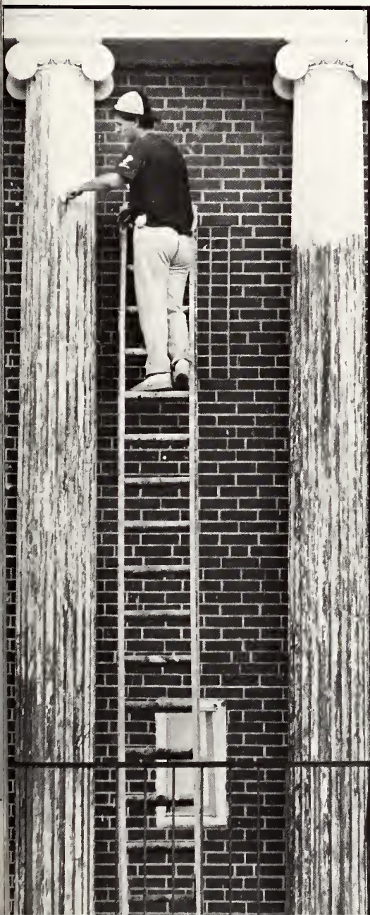
John Anderson brushes paint on the pillars at the Sigma Nu fraternity as part of a pledge project. (Photo by John LaBarge)
