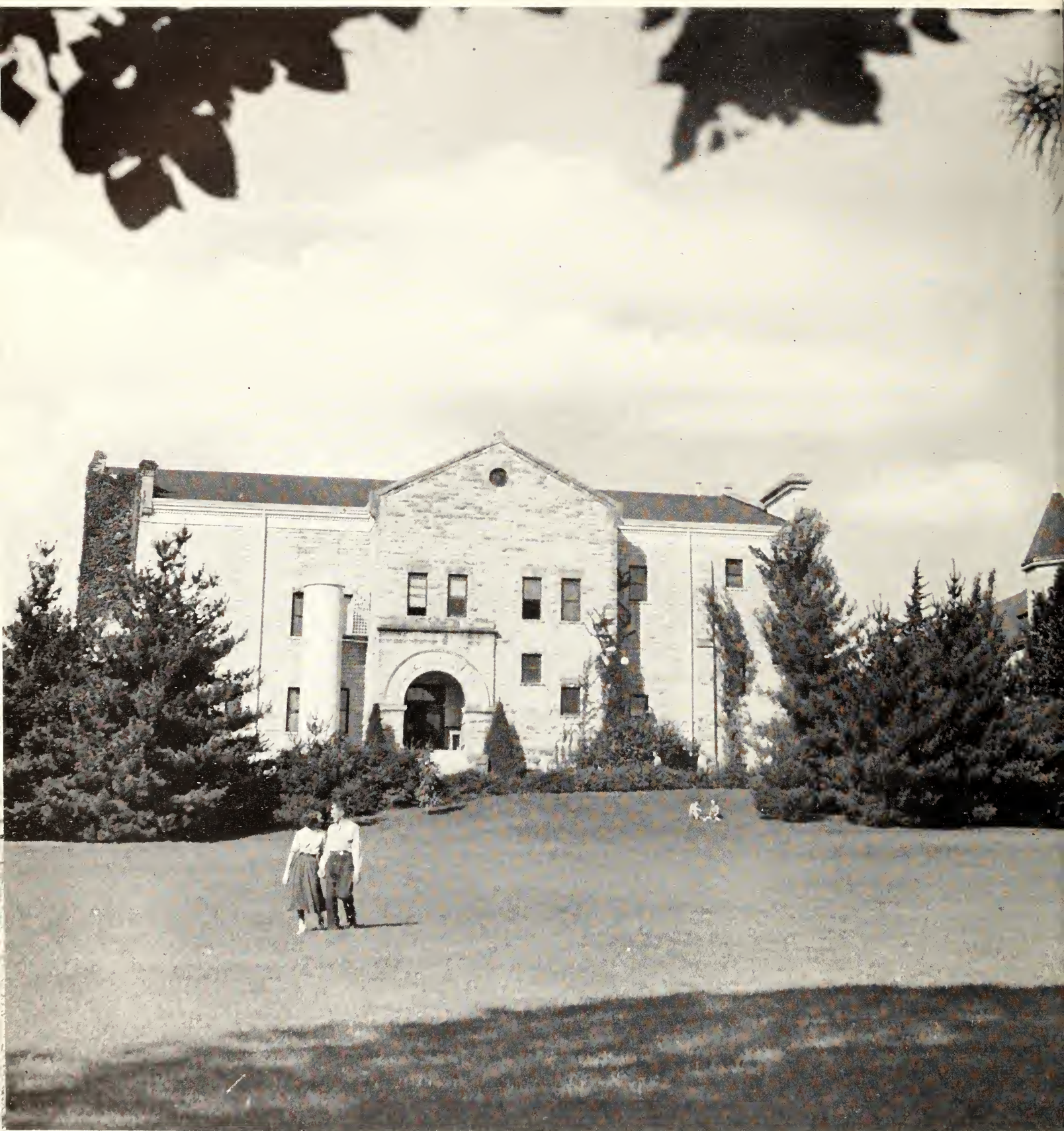
WALKING TOGETHER this carefree couple crosses the grassy turf sloping eastward from the auditorium. The seemingly austere auditorium with its obtrusive cylindrical, chute-type fire escape appears vacant though the photograph was taken when the structure was filled at assembly-time.
