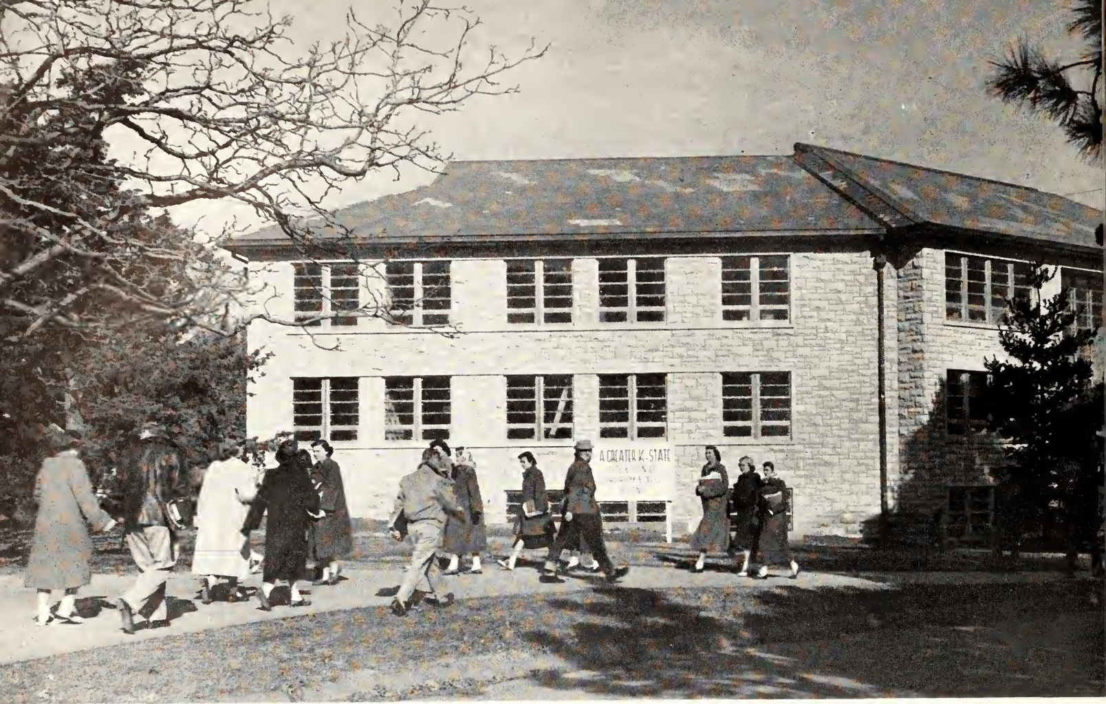
SPRING SEMESTER saw the offices of the Dean of Arts and Sciences, the departments of English, Speech, Modern Languages, and History, Government, and Philosophy move into the newly completed $655,000 K-State classroom building, east of Anderson hall.
