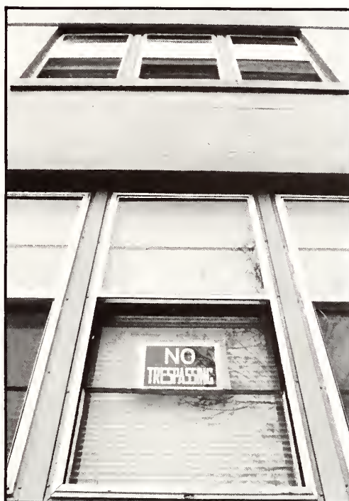
BECAUSE OF UPKEEP PROBLEMS the residence hall now stands empty. Plans were made for a new dormitory at K-State-Salina. (Photo by David Mayes)
