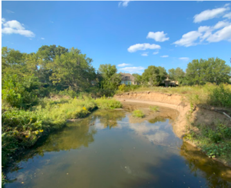
Creek Bank Erosion
