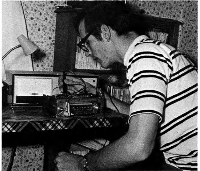
A tube tester, one of David's newest additions to his electrical equipment answers the question, "Is this tube a good one?"
