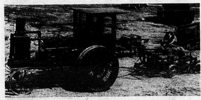
The first gang plows were on independent beams—this is the "Grand Detour" plow, pulled by the 20-40 kerosene-burning tractor of 1912.
