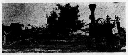
s an 1869 model "portable" steam engine operating an 1869 "Eclipse" thresher. The machine was in good running order, even the whistle.
