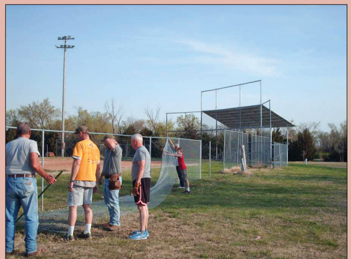
Installing the Potwin baseball field fence.
