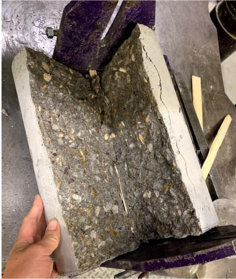
Figure 3-7 Cracked Cylinder - Tensile Splitting Test
