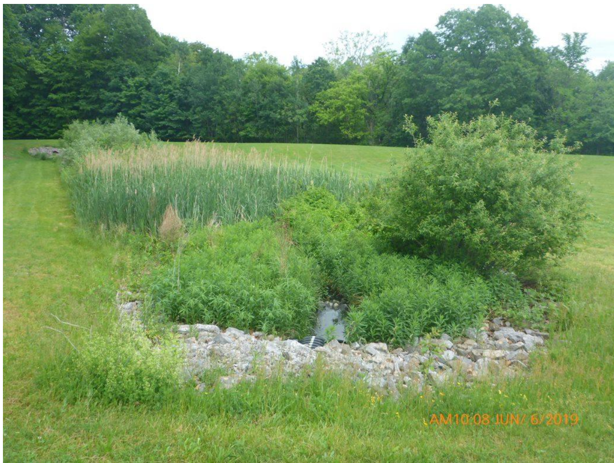
Appendix Figure B.3: Photo of a functioning vegetated filter strip with a stone-lined channel and dense native vegetation (Source: Steven Chase for USEPA, 2019, via EPA NPDES fact sheet)
