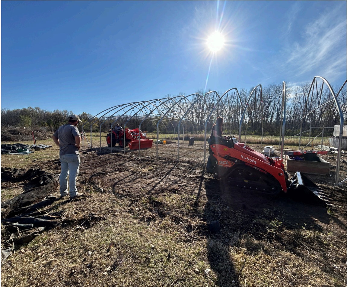
Figure 2.8: Willow Lake Farm high tunnel construction (Littlefield 2024).
