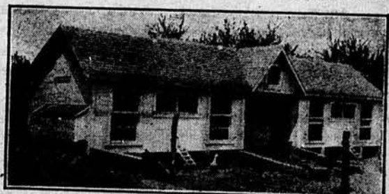
This Poultry House Has an Open-Front "Basement," Where Birds Seek Shelter From Storms and Bad Weather
