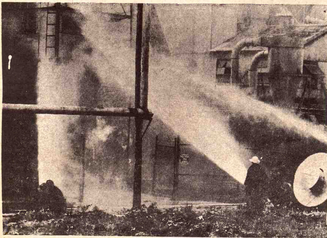
Hoses were trained on a large chamber called a desolventizer-toaster mounted outside the extractor plant. Firefighters were able to extinguish a fire in and below the toaster by spraying water over the machine and lowering the temperature of the vapor and liquid inside. Firefighters estimated that 1.3 million gallons of water were used in controlling the fire.
