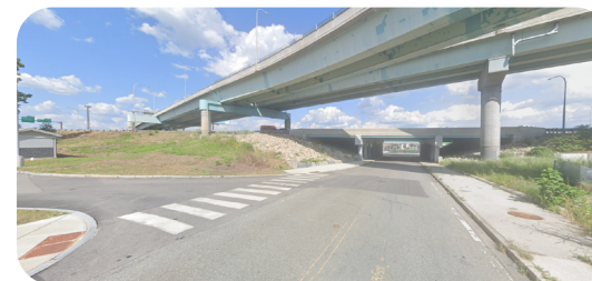
Figure 5.44 | Existing Conditions of Blackstone St. Near I-95
