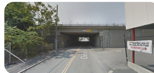
Figure 5.57 | Existing Conditions of Oxford St. Underpass
