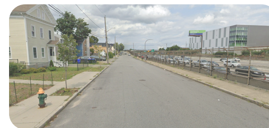
Figure 5.40 | Existing Condition of Byfield Street
