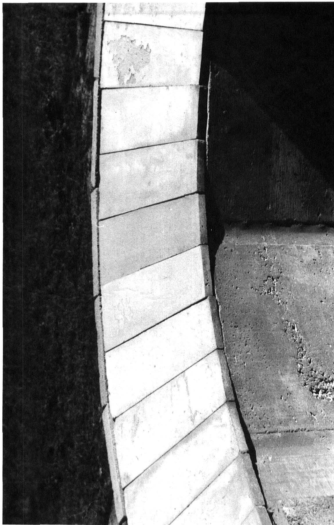
Plate 2-2. The concrete collimator blocks in position on top of silo wall.
