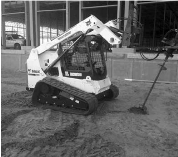
Figure 2-5: Skid-Steer Installing Helical Ground Anchor (Reproduced from Dayton Superior, 2017)
