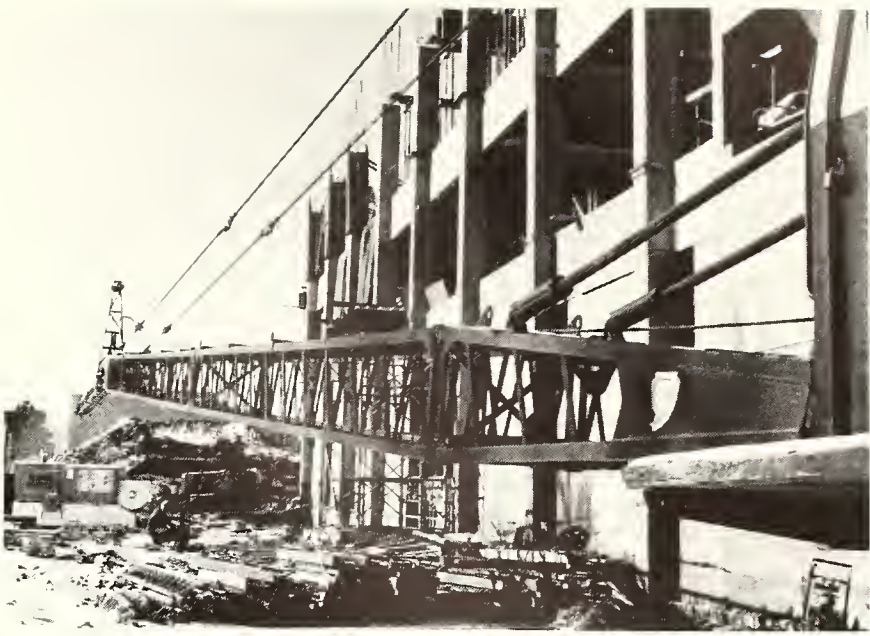
Pieces of massive earth-moving equipment are located at the site of the new biological sciences building.
