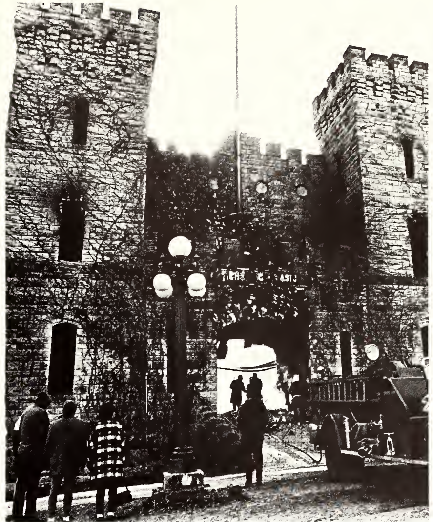
While portions of the gutted gym continue to smolder, officials investigate the site for signs of arson.
