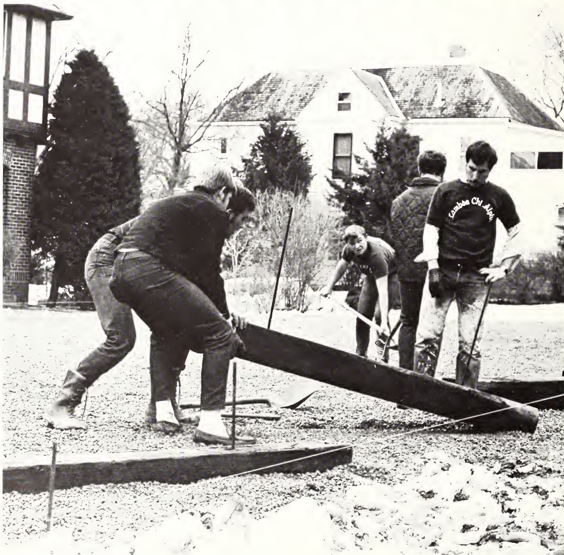
In order to complete their requirements for initiation, Lambda Chi pledges install parking dividers.
