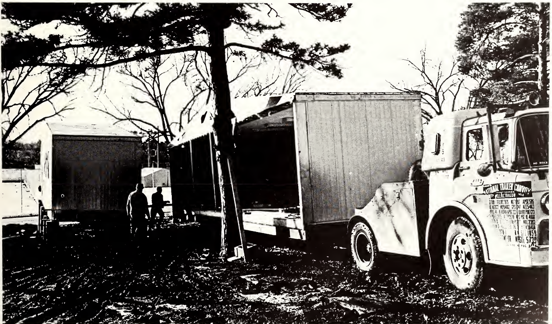
Music classrooms destroyed in the fire were replaced by five trailers acquired from Washburn University.
