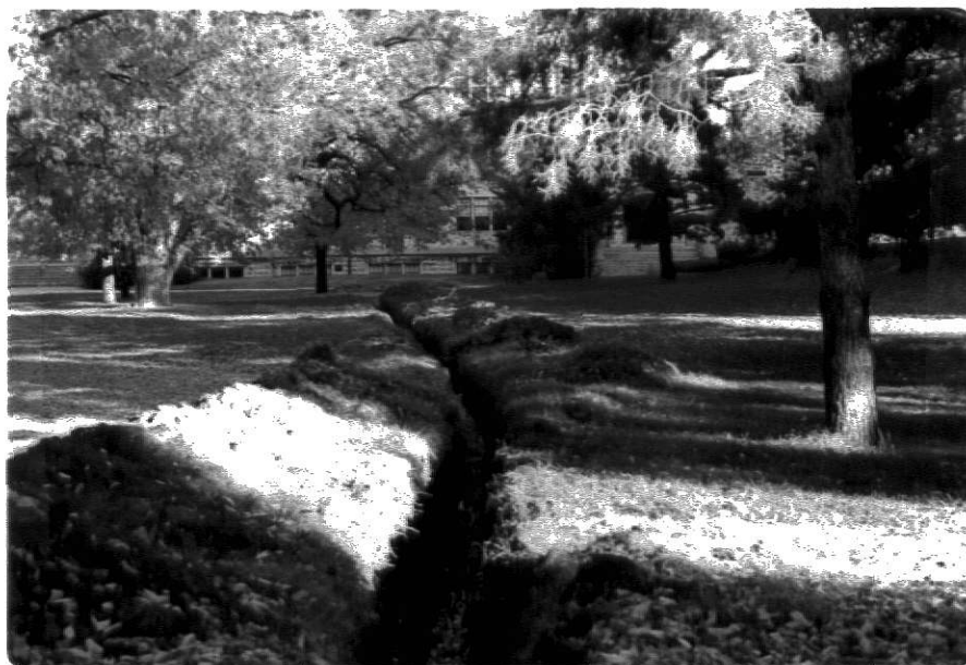
Maintenance and Construction (October 1972)
