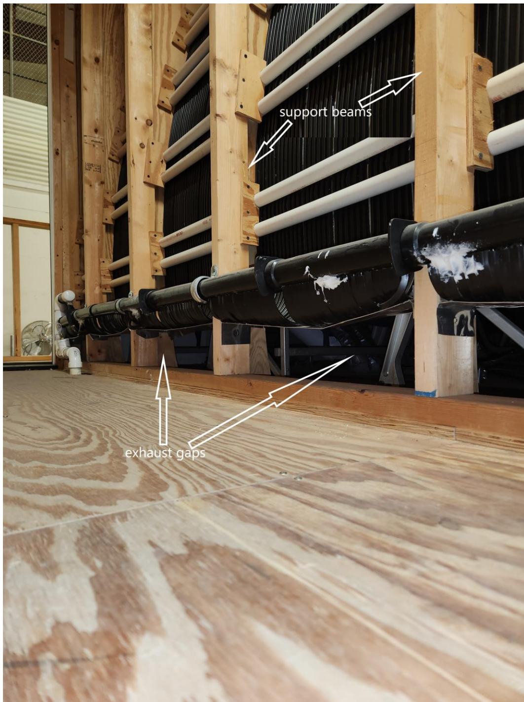
Figure 3.3: Support Columns and Exhaust Gaps
