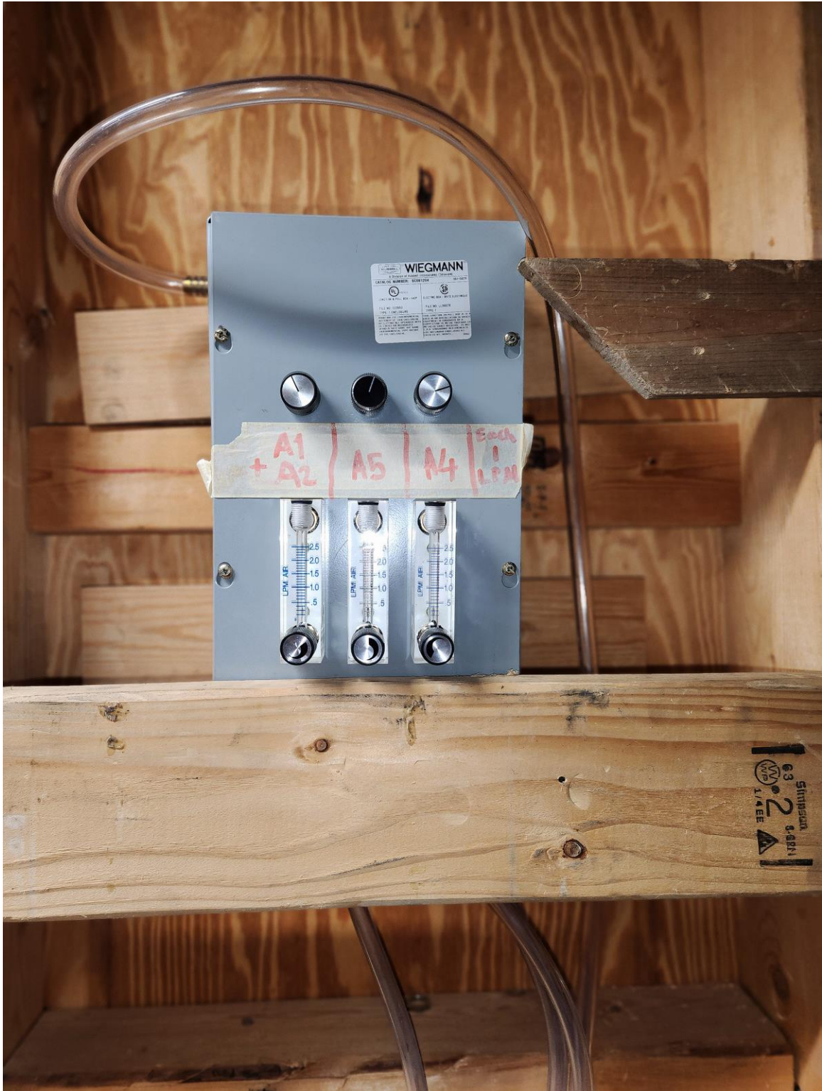
Figure 3.23: Flow Balancing System
