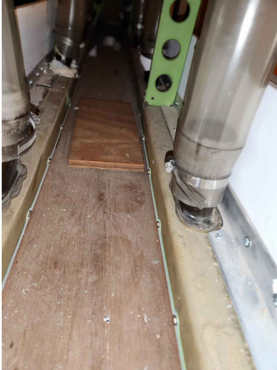
Figure 3.12: Connections to Linear Diffuser
