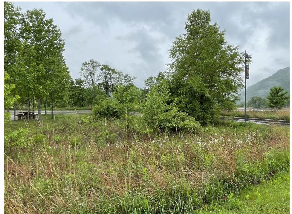
Figure 10 Sandstone Visitor Center Naturalized Detention Basin, Skabelund 2022
