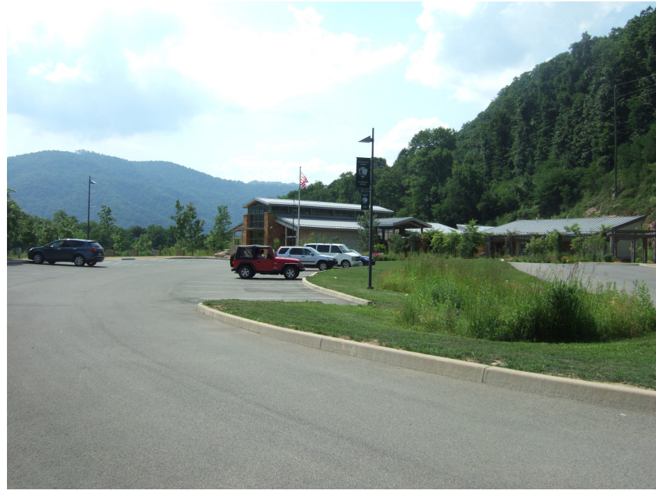
Figure 8 Sandstone Visitor Center Bio-Swale, Skabelund 2022
