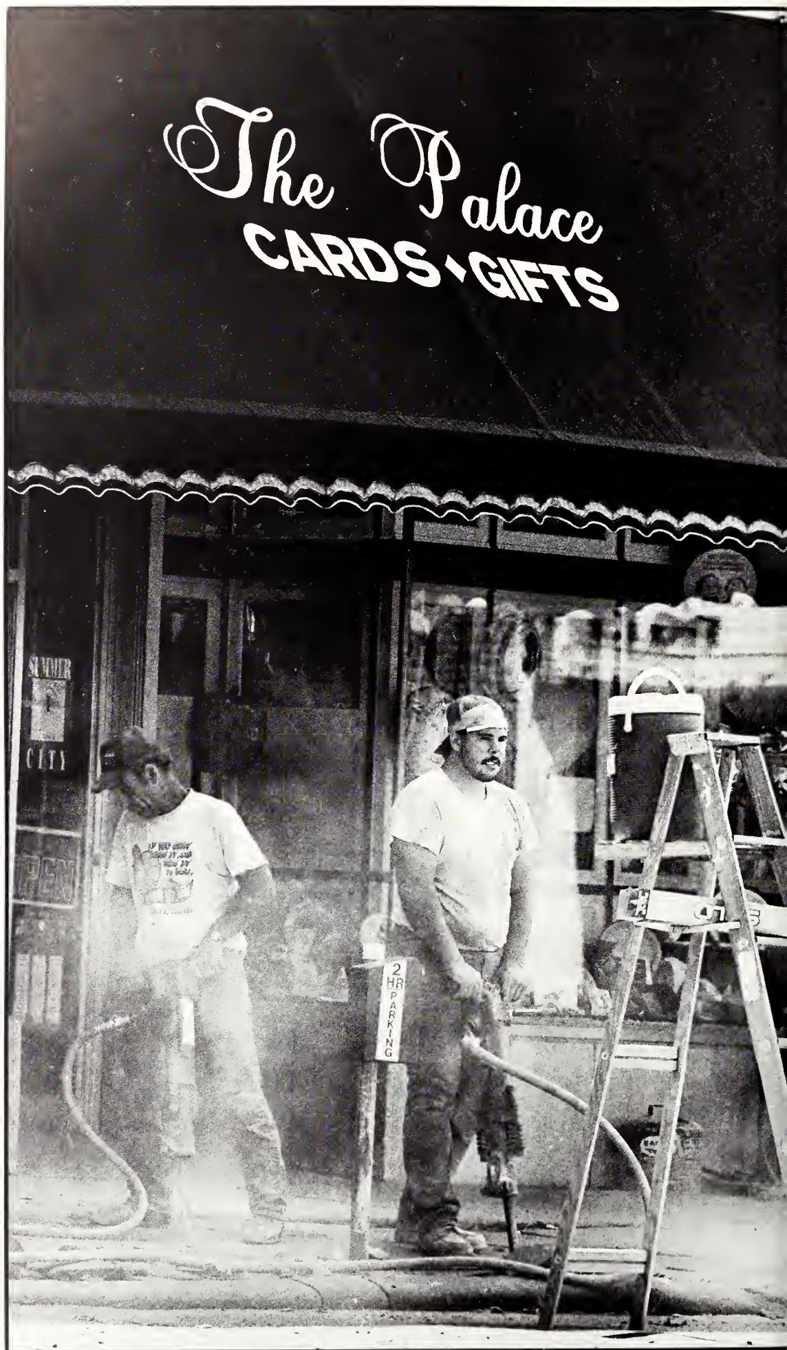
◆ Leo Jensen, left, and Mike Volanti, Cherney Construction, Manhattan, begin the $1.95 million renovation of Aggieville by tearing up sidewalks. (Photo by Christopher T. Assaf)
