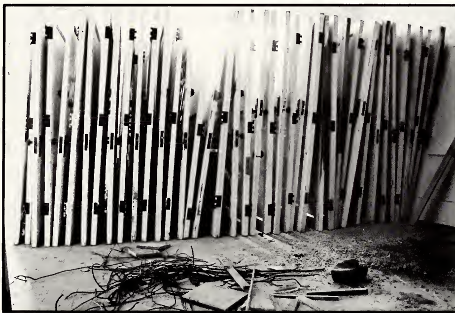
♦ Doors from individual rooms are stacked together on the first floor of Van Zile Hall while the rooms are repaired. (Photo by Steve Wolgast)
