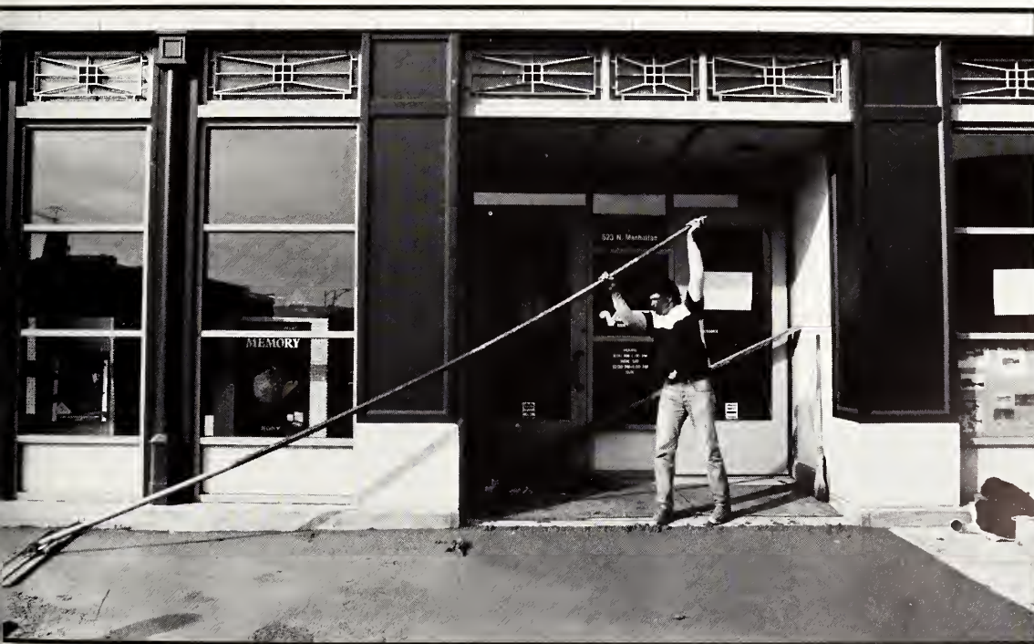
◆ Al McKee trowels concrete for the resurfacing of the Aggieville sidewalks. (Photo by Oliver Kaubisch)
