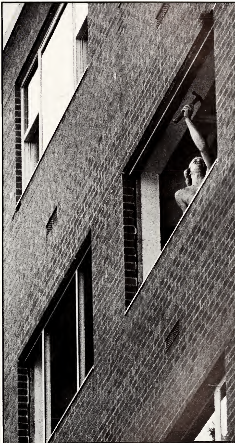
◆ Randy Miller, of Window Systems Construction, hammers a new window frame into place in Goodnow Hall. All windows in the residence hall were replaced in July and August before classes resumed. (Photo by Christopher T. Assaf)
