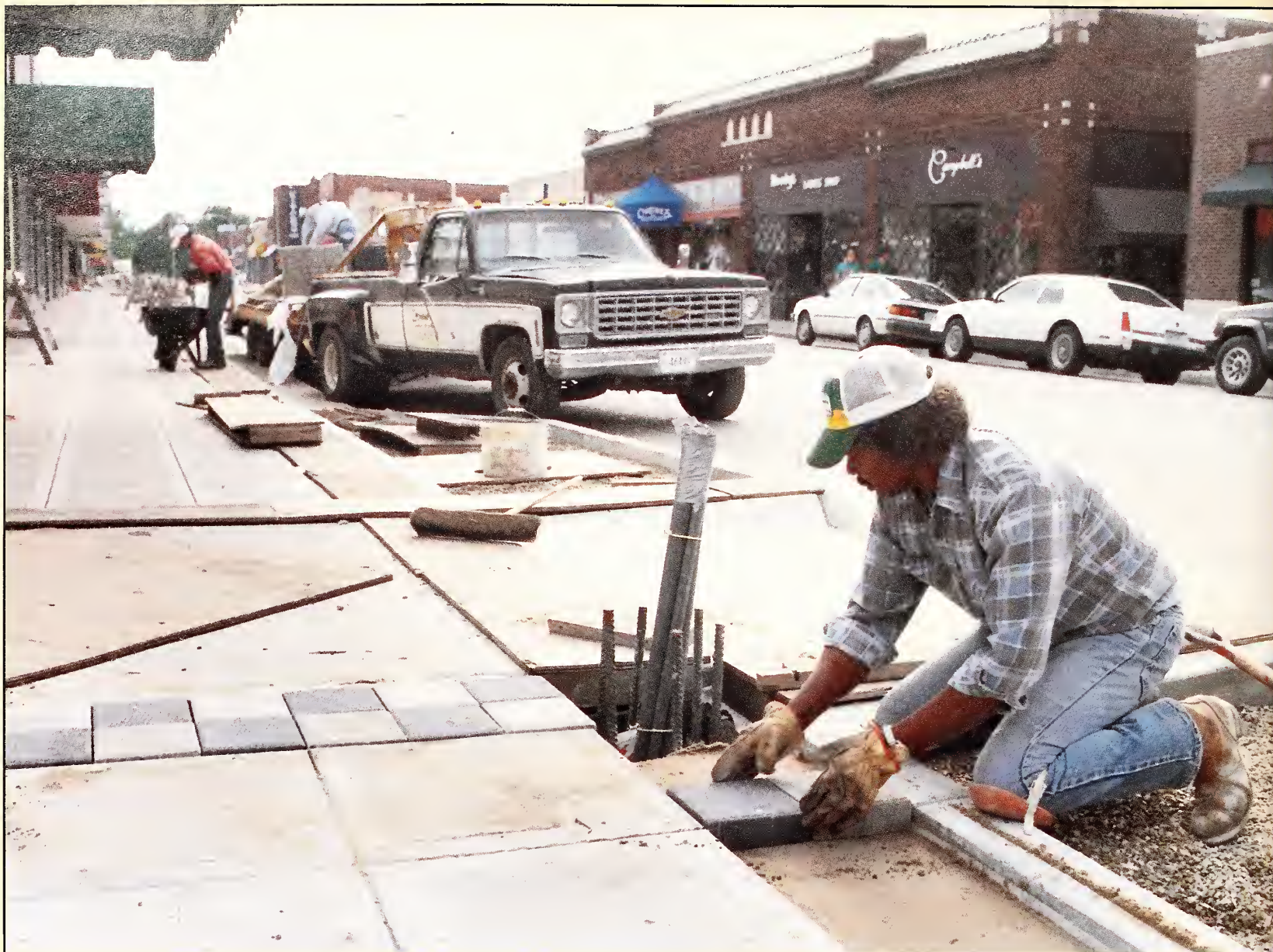
◆ Charles Alexander of Cheney Construction Inc. lays down paving bricks along the new sidewalk in Aggieville, one of the many improvements being done. (Photo by Brett Hacker)
