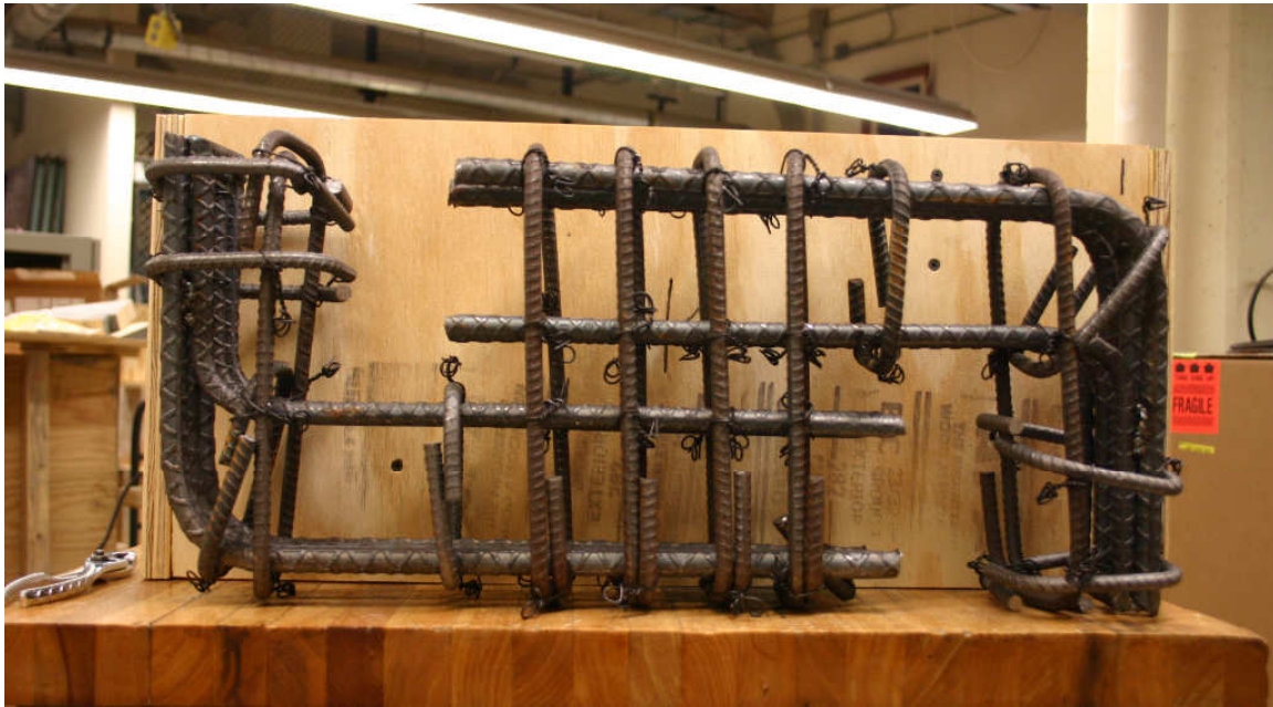
Figure 7.4: Completed Rebar Cage
