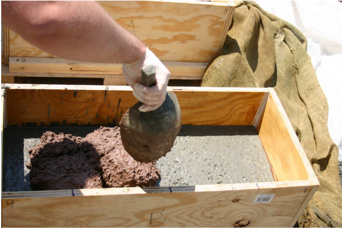
Figure 6.4: Concrete Placement for Small Core Block
