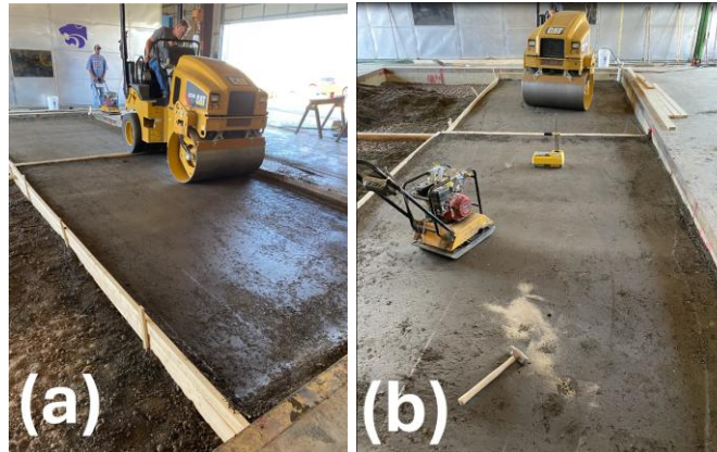
Figure 5.12 SFDR Base Construction
