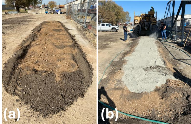
Figure 5.10 FDR Materials: (a) with 2% Soil; (b) Cement
