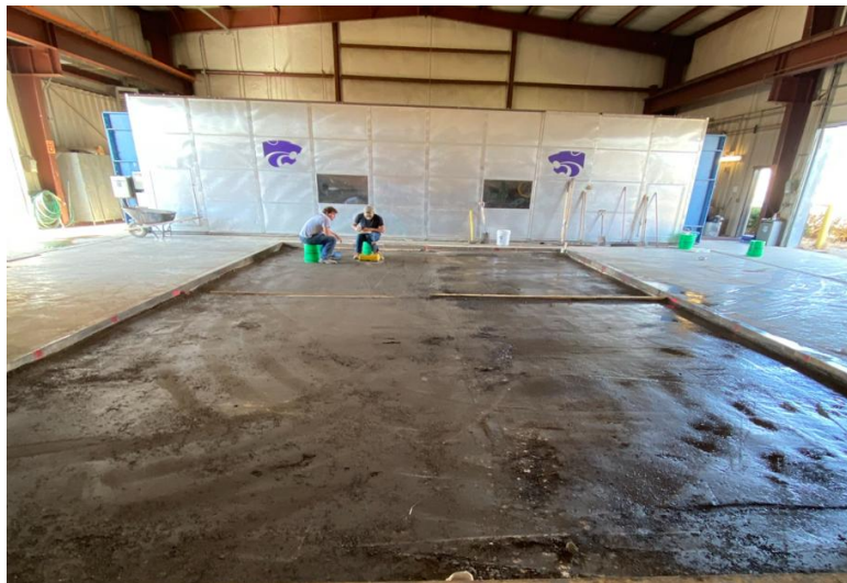
Figure 5.13 Nuclear Gauge Testing on Compacted SFDR Base
