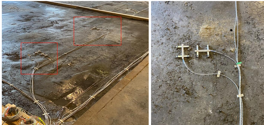
Figure 5.21 H-Bar Strain Gauge Installation
