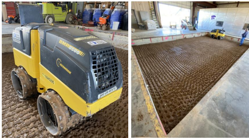
Figure 5.6 Soil Compactor and Compacted Layer
