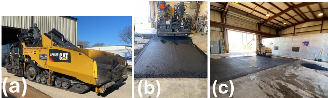
Figure 5.15 (a)HMA Mixture Paver; (b) Paving; (c) Compaction
