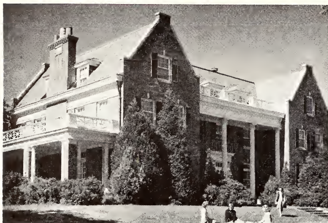
The Kappa Chapter house is located at 517 North Delaware.
