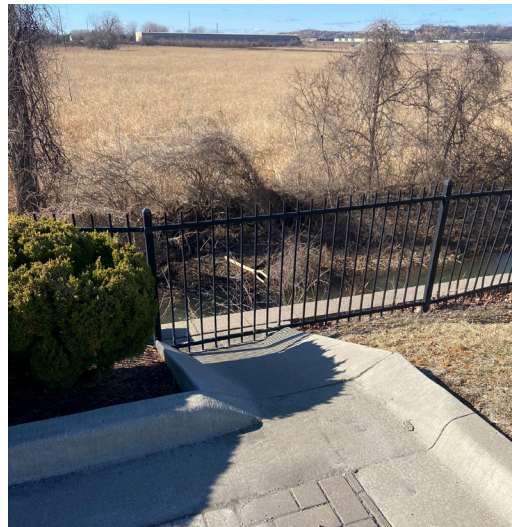
Figure 1.6 Picture of concrete swale at The Landing at Briarcliff in Kansas City, Missouri (Brizendine, 2022).
