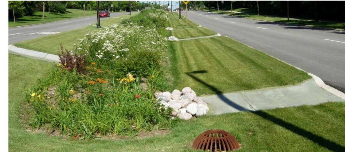
Figure 1.3 Picture of a bioswale between roads (Volkening, 2023).
