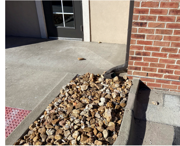
Figure 4.10- Infiltration trench at the landing at Briarcliff (Brizendine, 2023).
