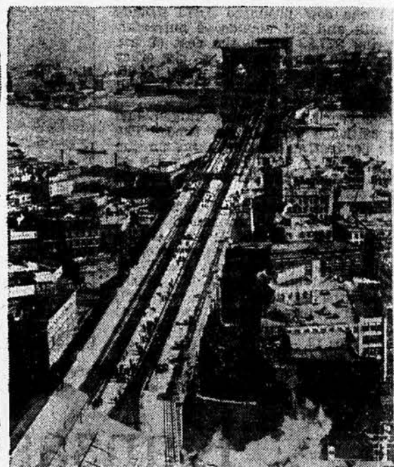
Old Brooklyn Bridge Nearly 40 Years Old Shows Its Infirmities; Giant Cables Slip But Engineers Say It is Still Safe and Will Last for 100 Years or More
