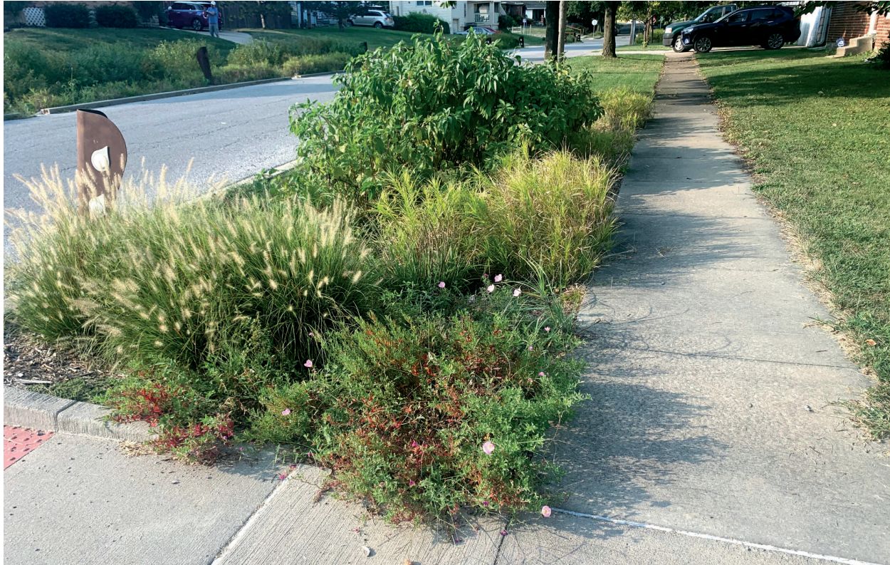
Figure 38: Orderly Planted Right-Of-Way Bioswale
