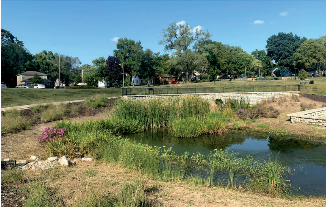
Figure 9: Wetland Pond at 81st Street & Troost Avenue.
