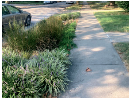
a (Bottom Left): Green Stormwater Infrastructure 17
