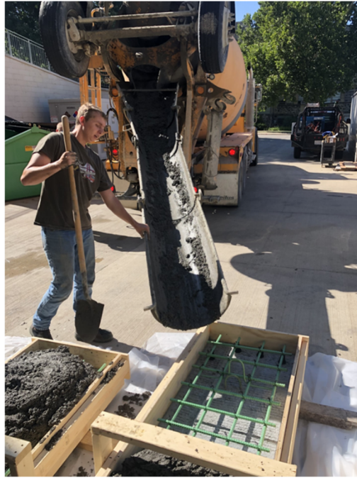
Figure 18: Placing of Topping
