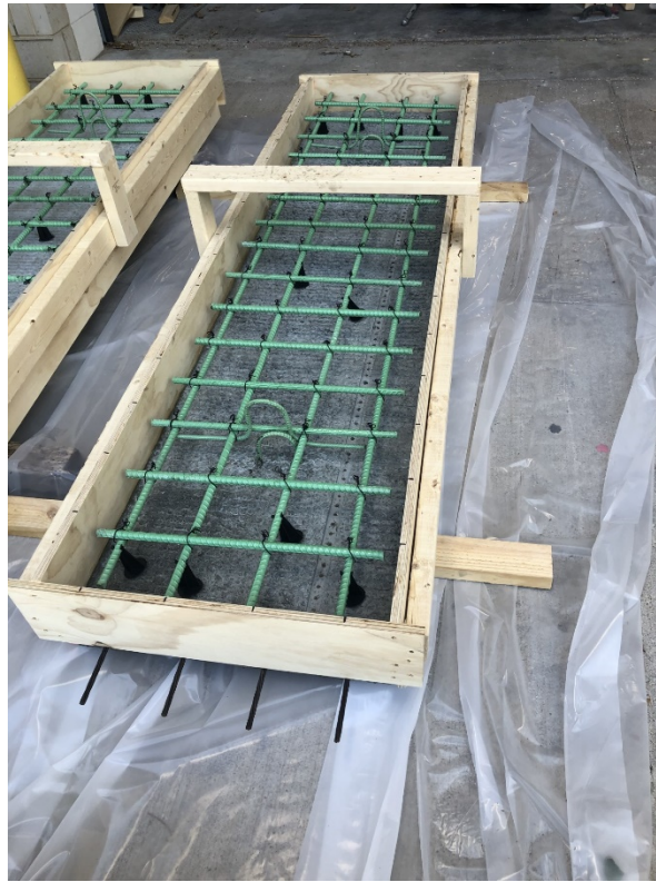
Figure 17: Topping Form and Placed Rebar
