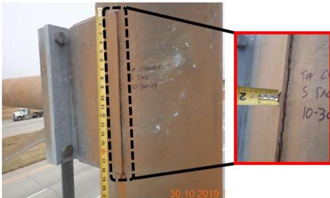
**Figure 5.13 Crack in the weld toe in Sedgwick structure, courtesy of KDOT (Bureau of structural and geotechnical services).**
