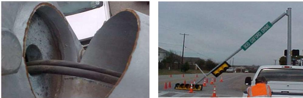
**Figure 1.2 Fatigue failure at mast arm connection of traffic signal [4]**
