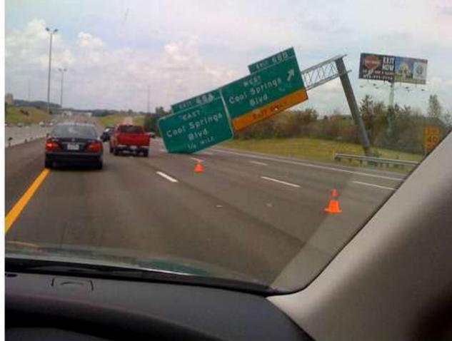
**Figure 1.1 Failure of cantilever sign support structure along I-65 in Tennessee [3]**
