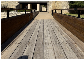
Fig. 4.23 Wood decking (Goold 2025)
