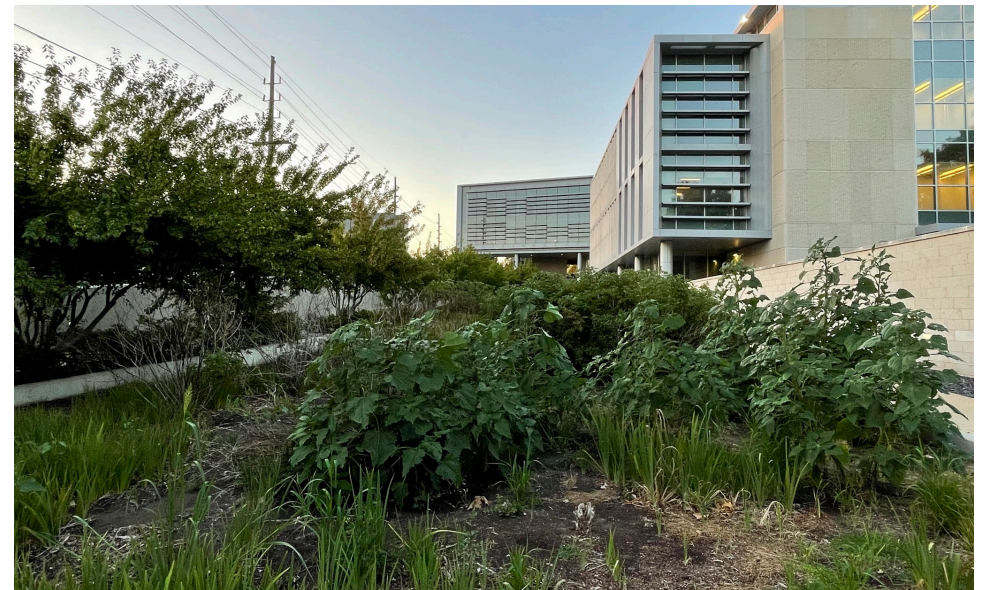
Fig. 3.37 Tall unflower moves into lowest bioretention cell (Skabelund 2023)
