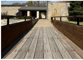
Fig. 4.23 Wood decking (Goold 2025)
