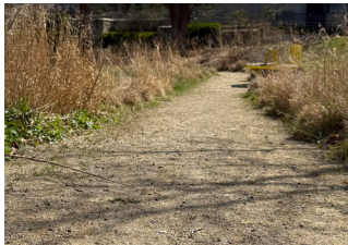
Fig. 4.19 Crushed limestone (Goold 2025)
