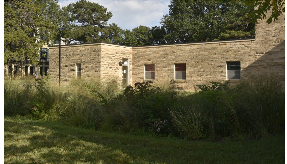
Fig. 3.20 New bioretention basin (Goold 2024)
