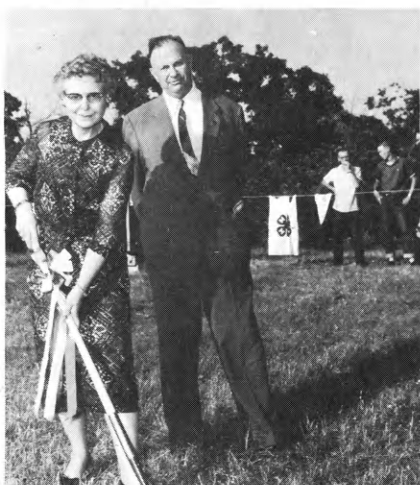
Mr. and Mrs. Ray Garvey break ground for the Asa Payne Cottage at RSR in 1958.
