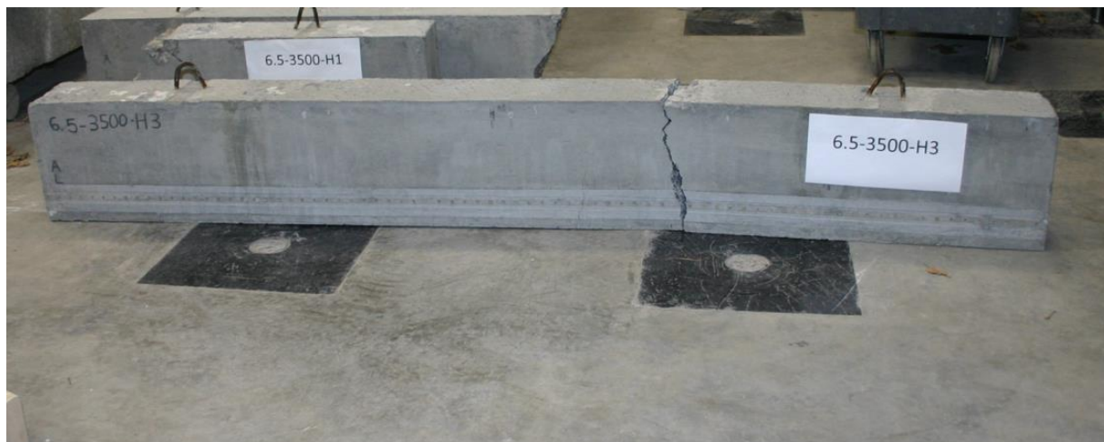
Figure D.8: Broken Beam Failing Through Strand Rupture.
