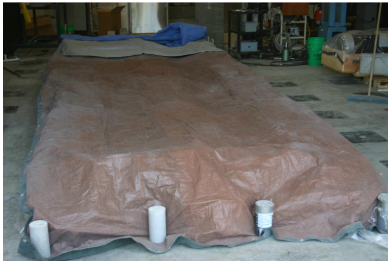
Figure 3.11: Covered Beams During Concrete Curing.
