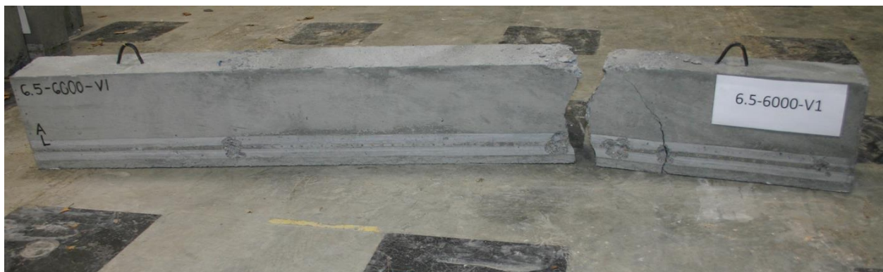
Figure D.49: Broken Beam Failing Through Strand Rupture.
