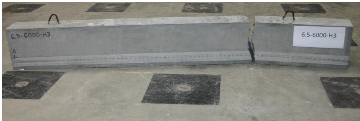
Figure D.43: Broken Beam Failing Through Strand Rupture.
