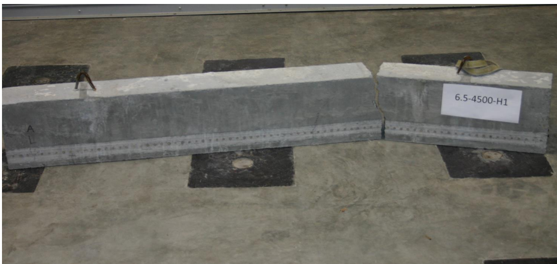
Figure D.19: Broken Beam Failing Through Strand Rupture.
