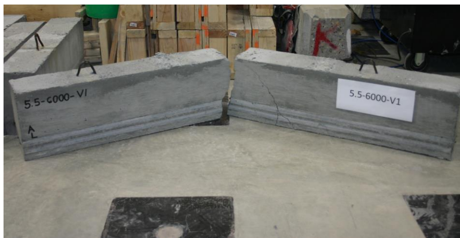
Figure D.47: Broken Beam Failing Through Strand Rupture.
