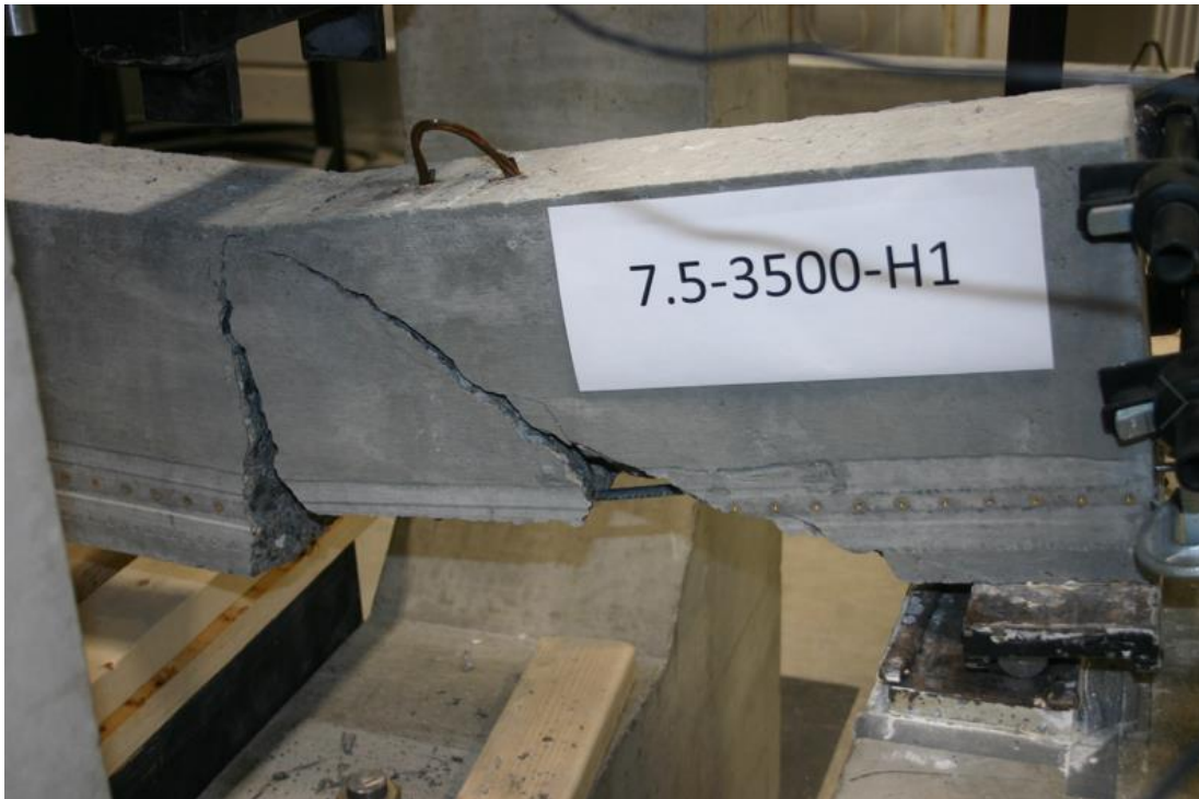
Figure 4.18: Full Development of Flexural-Shear Crack Shown After Failure of Specimen.
