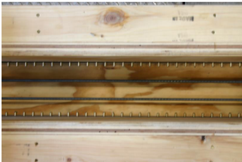
Figure 3.12: Top of Formwork Showing Prestressing Wire and Brass Inserts Spaced at One Inch on Center.
