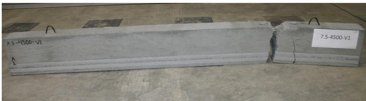
Figure D.33: Broken Beam Failing Through Strand Rupture.
