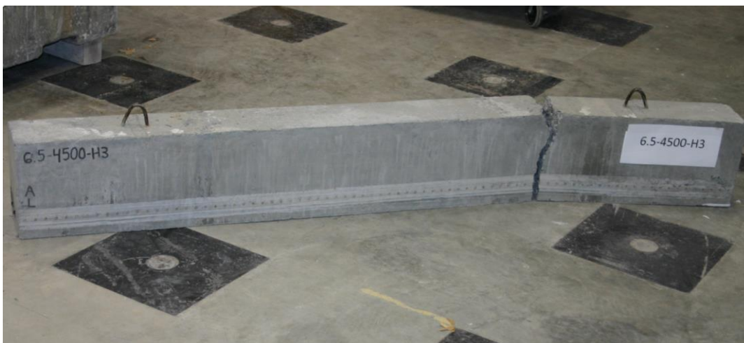
Figure D.25: Broken Beam Failing Through Strand Rupture.
