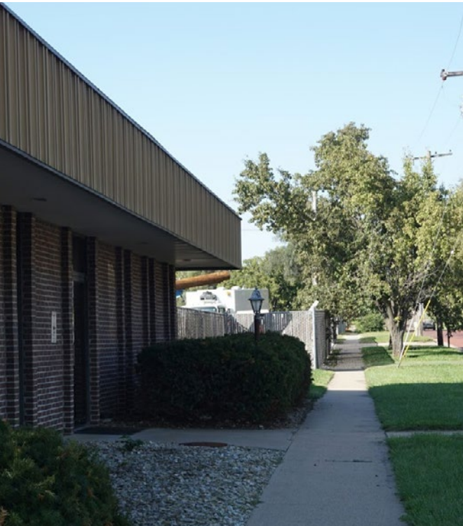
Figure 2.5.8. Original UP Depot looking West (Belanger, Blake. 2019. Depot from the East. Photograph.)
