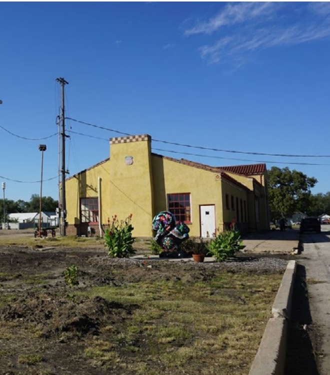
Figure 2.5.6. Original UP Depot looking West (Belanger, Blake. 2019. Depot from the East. Photograph.)
