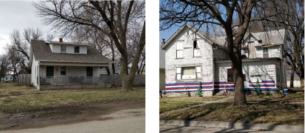
Figure 3.5.4 Examples of housing in Southwest Marysville The Southwest Marysville neighborhood has a diverse mix of housing quality. The home on the left represents a good quality structure, and the structure on the right is dilapidated.
