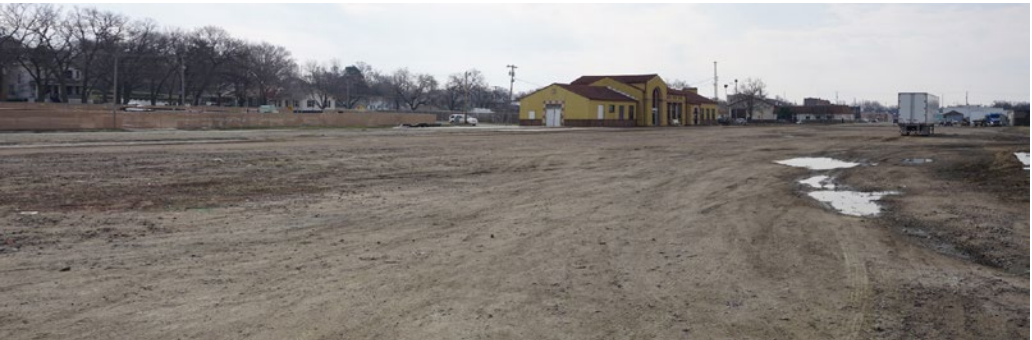
Figure 2.1.2 Much of the Union Pacific Depot site is undeveloped Gravel lots and unmaintained vegetation surround the building. (Belanger 2019)
