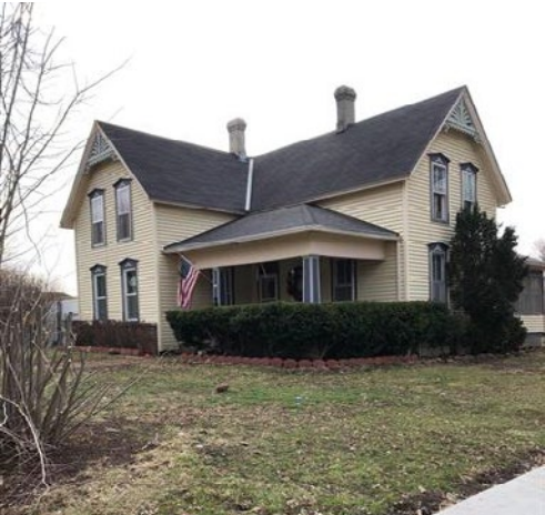
Figure 3.4.17 (Top Left) Sound Condition Example of a home considered of sound condition. (Geist, 2019)
