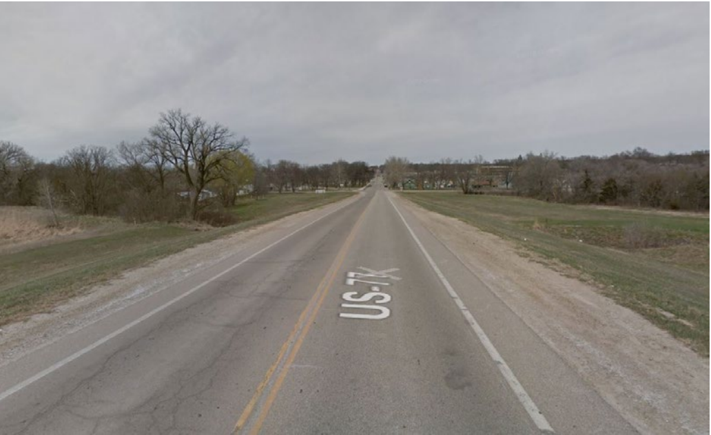
Figure 1.4.3 US 77 Highway This highway transitions into 10th Street in Marysville and is one of the main roads into the town. (Google 2019)
