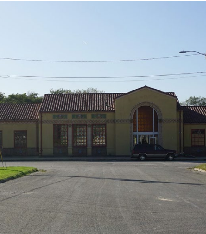
Figure 2.5.5. Original UP Depot looking West (Belanger, Blake. 2019. Depot from the East. Photograph.)
