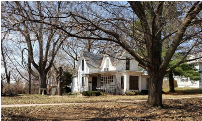
Figure 3.2.11 Older Home Located in the southern portion of the neighborhood on N 11th St., this is an example of an older home that needs refurbishment.
