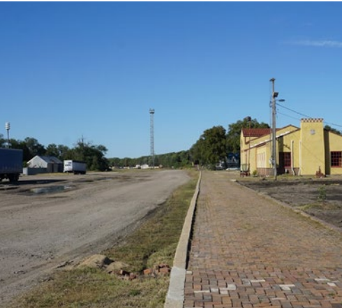
View looking North of the site. The brick platform is run down and needs to be releveled.
