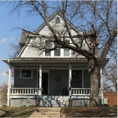
Figure 3.3.16 Minor Rehabilitation: A dwelling unit that shows signs of multiple deferred maintenance, or that requires the repair of one major component.
