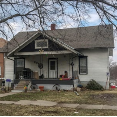
Figure 3.3.17 Moderate Rehabilitation: A dwelling unit that requires multiple repairs and the replacement of a major component.
