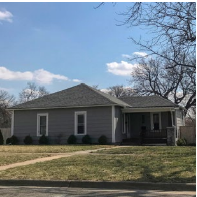
Figure 3.3.14 Excellent: A dwelling unit that is new or well maintained and structurally intact (no visible deficiencies). Foundation appears structurally undamaged, and roof-lines are straight. Windows, doors, and siding are in good repair. Exterior paint is in good condition.
