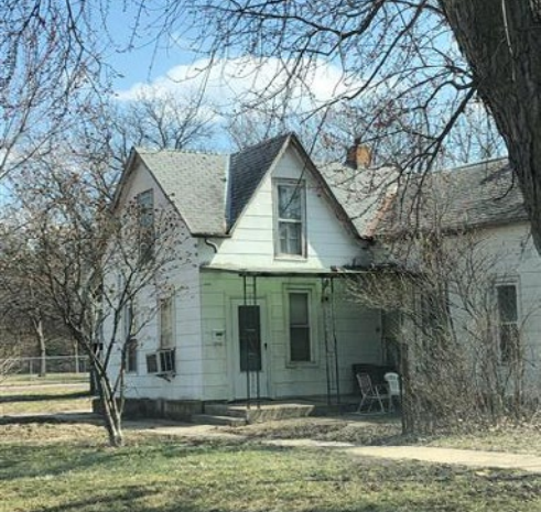
Figure 3.4.19 (Bottom Left) Moderate Rehab. Condition Example of a home considered to be of moderate rehabilitation condition. (Frohberg, 2019)
