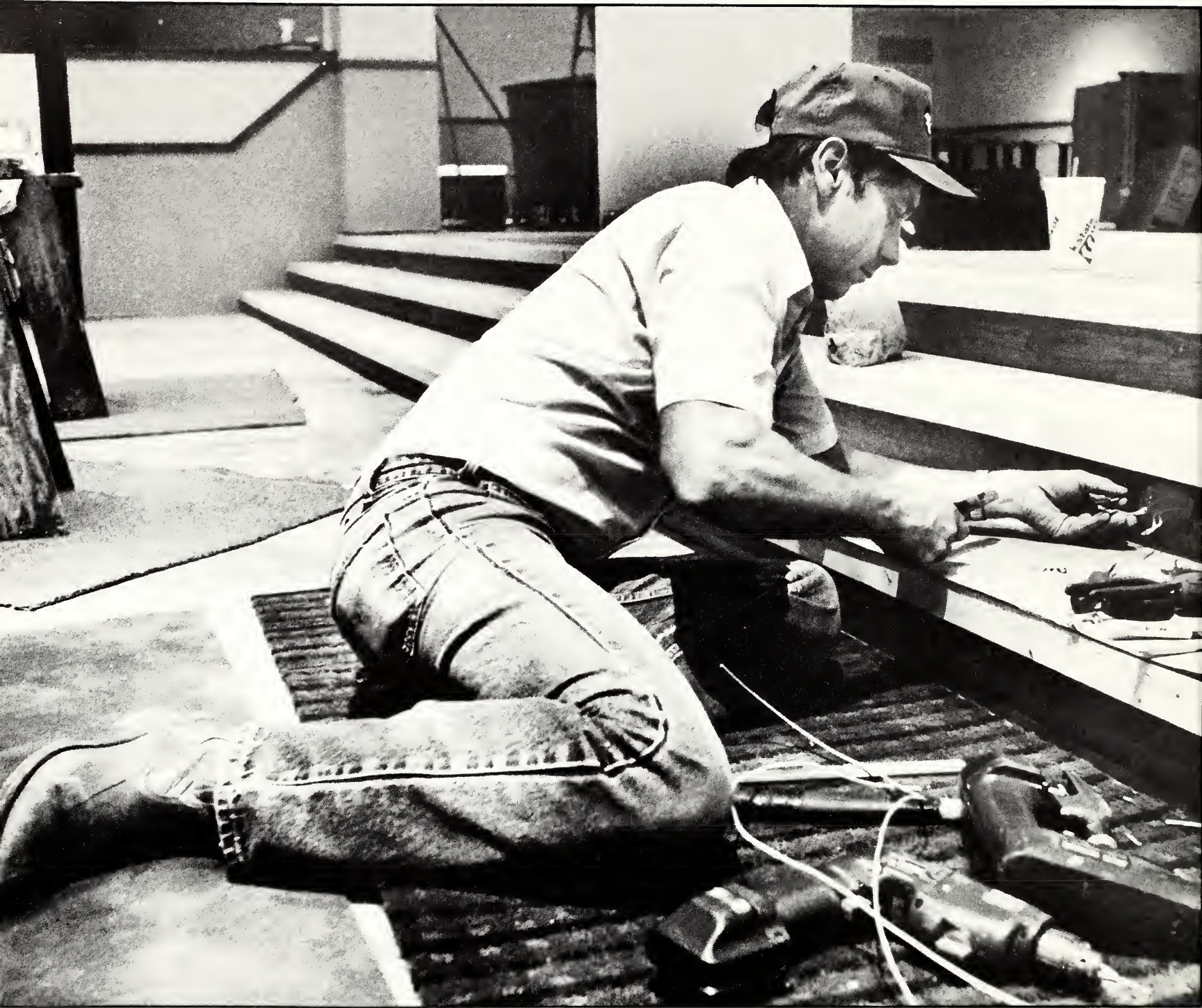
Union Station's electrical wiring system gets finishing touches from Steve Hemphill, Wamego. A three-day program of activities kicked off the Union's newest social offering. (Photo by J. Kyle Wyatt)
