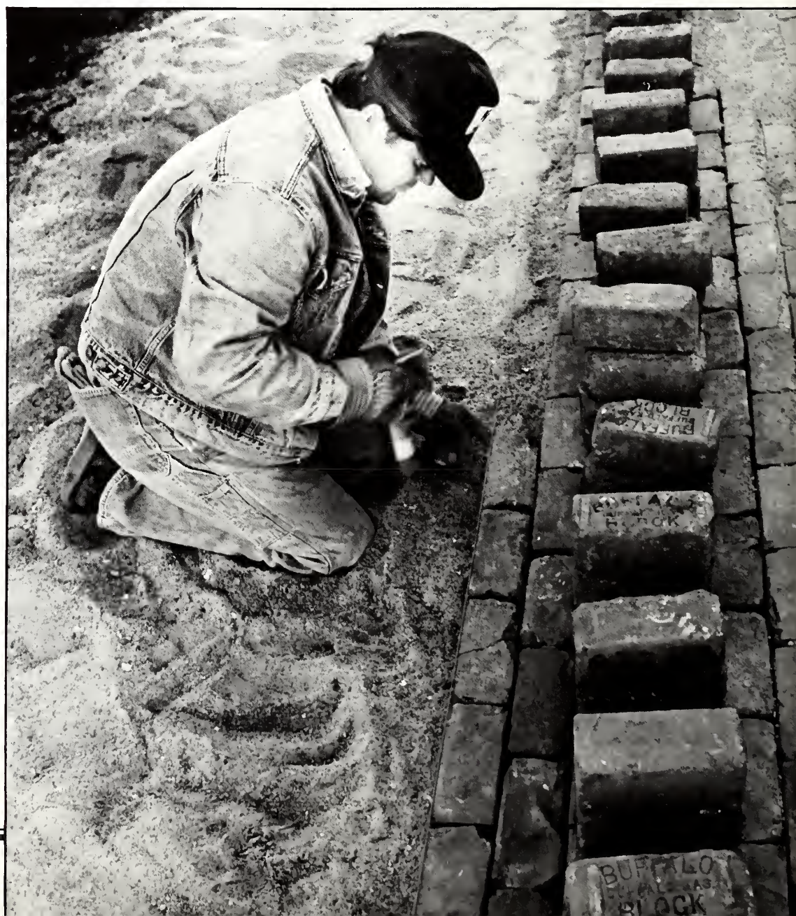
Michael Reasoner, facilities and grounds maintenance worker, lays bricks for a bicycle parking area in front of Fairchild Hall. His was one of many remodeling projects around campus. (Photo by Mike Welchans)
