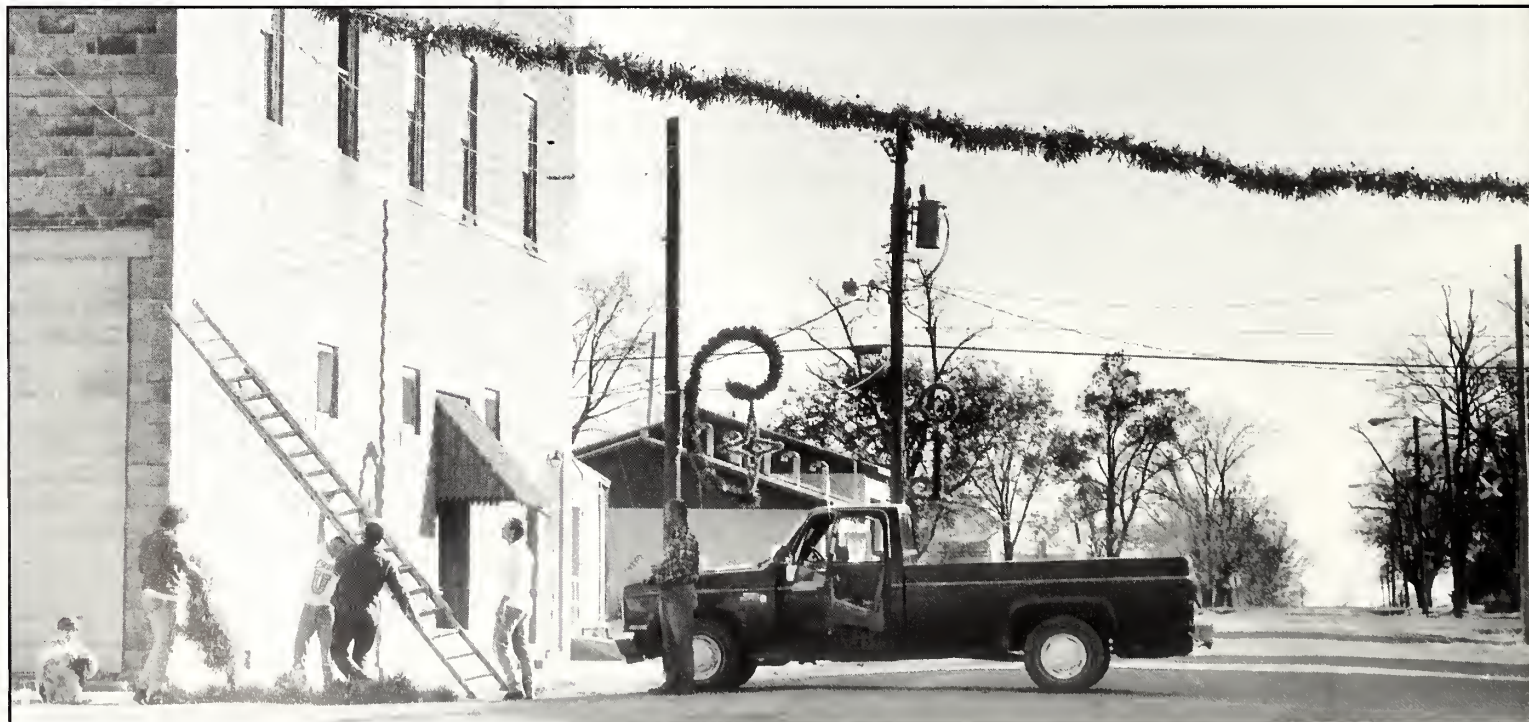
T ownspeople work with S.A.V.E. volunteers to string garland over the intersection of Third and Main Streets. During the project they discovered a manual elevator in the old mortuary building. (Photo by Brian W. Kratz)
