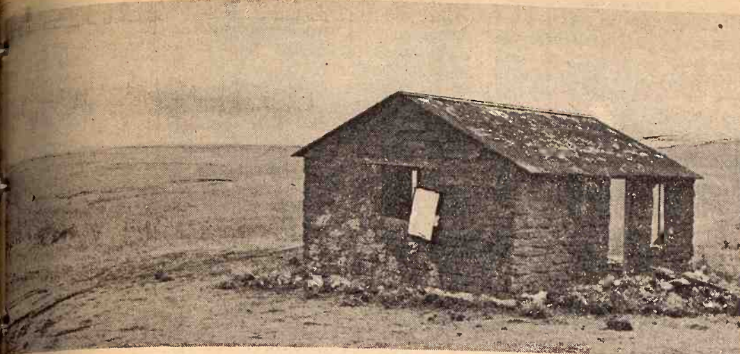
FIBERGLASS SODDY This sod shanty in the Flint Hills of Chase county looks as if it might be something abandoned 80 years ago, but it's really a mud-plastered fiberglass construction used for the filming of "Bad Company," a Paramount movie which has used the Flint Hills around Elmdale, Severy, and Neosho Rapids as a setting for shooting the past eight weeks.
