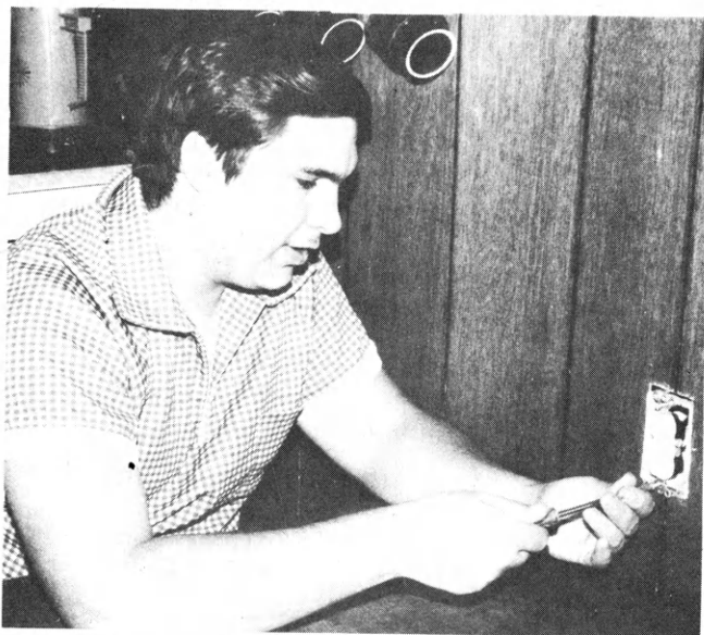
To provide a convenient place to plug in the toaster, Joe installs an electric outlet by the kitchen table.
