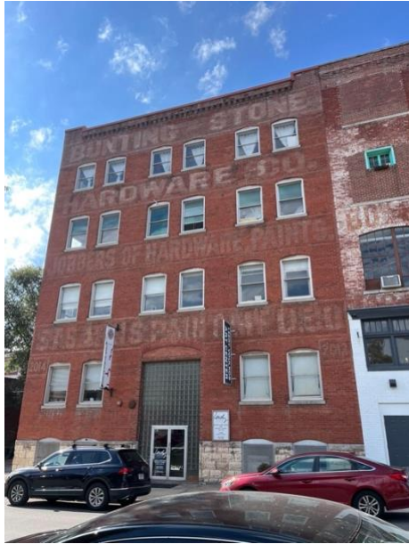
Figure 17. Example of Adaptively Reused Building in the Crossroads. John Pileggi, 2023.
