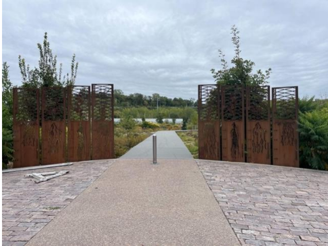
Figure 30. PPP Stormwater Retention & Trail West Bottoms. John Pileggi, 2023.
