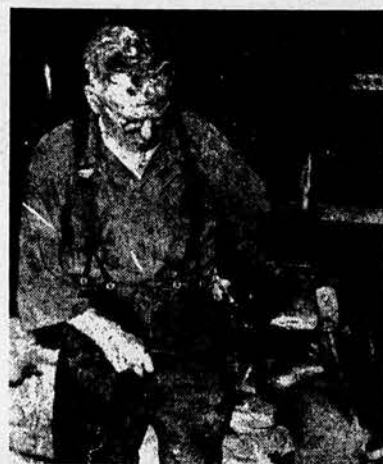
A homemade trip hammer does the shaping on a plowshare in the Bennett shop. Mr. Bennett is still active at 73 and personally rebuilt his shop after it burned in 1946.
