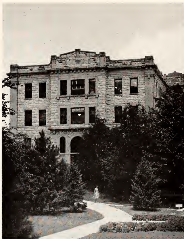
EAST WATERS HALL will soon be joined to West Waters by a connecting wing under construction this year. Most of the wing will be used for offices.
