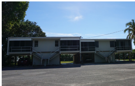
FIGURE 4.39: Staff Housing Area
