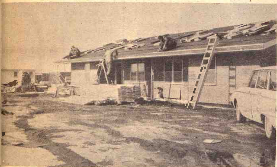
Roofing starts on one of the multi-unit dwellings.
