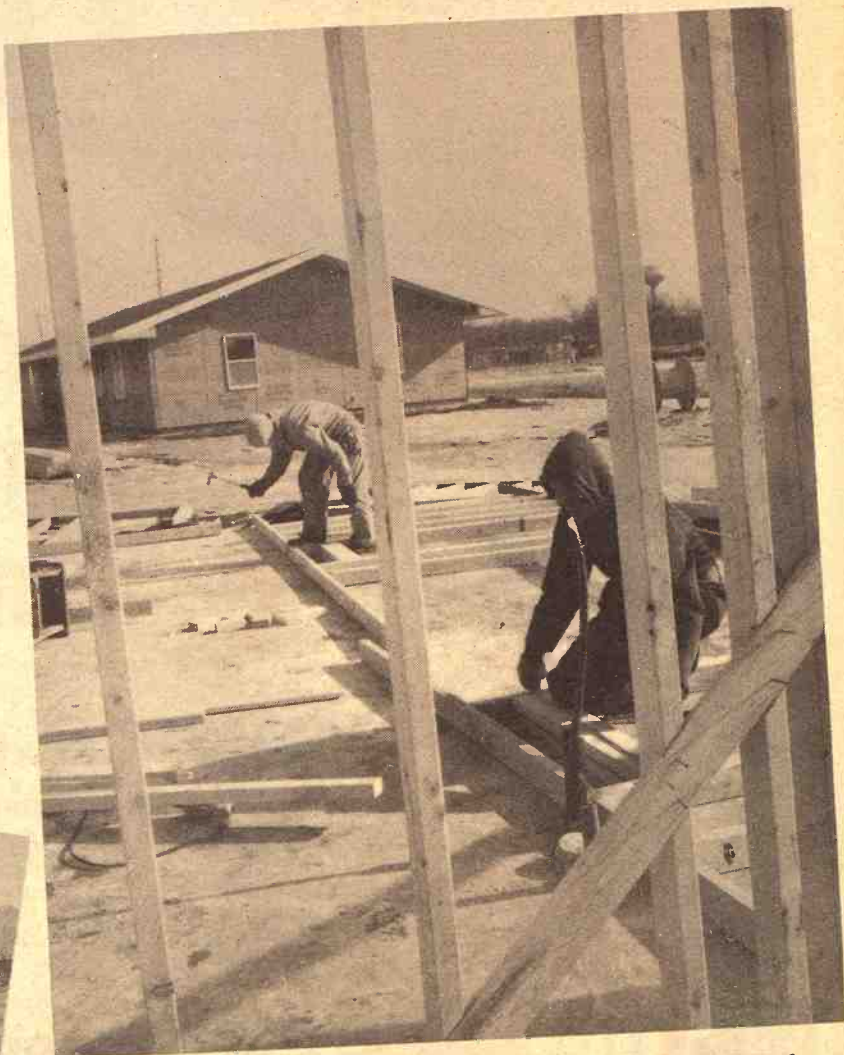
George Nemechek and Cecil Whiting of Blue Rapids assemble a wall frame.
