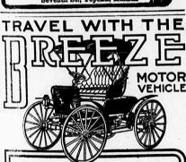
MODEL "J 650" Shown above, equipped complete with lamps, horn, rubber apron, full fenders, 1½" solid rubber motor tires and roller-bearing axles. Price, \$625.00.
