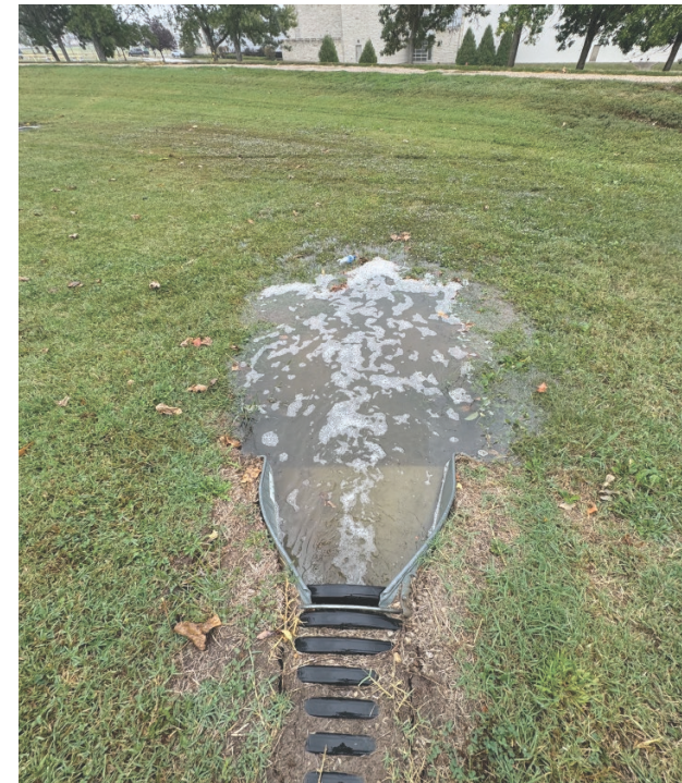
Figure 2.12 Northwest Outlet Pipe During Rain Event (Freelove 2024).
