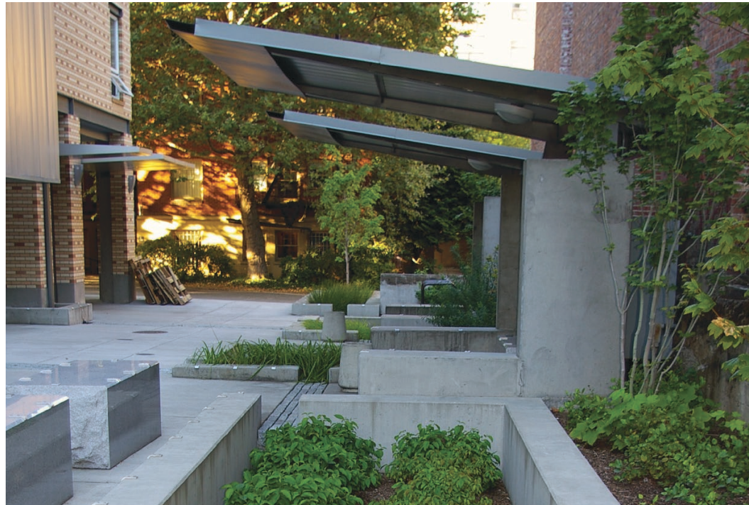
Figure 3.18 View of Green Infrastructure Connections at Stephen Elper Hall (Echols 2004). Used with permission.
