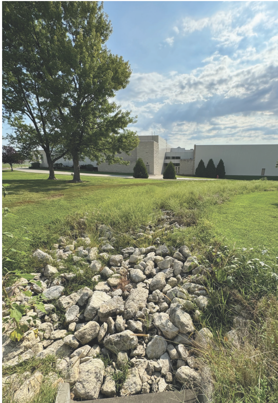
Figure 2.08 Existing Channels on the West Side of the Recreation Complex are Filled with Rock (Freelove 2024).
