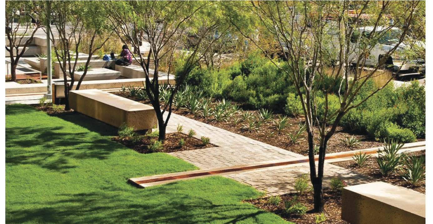
Figure 3.23 Steel Covered Runnels (Barbe & Ten Eyck Landscape Architects n.d.). Used with permission
