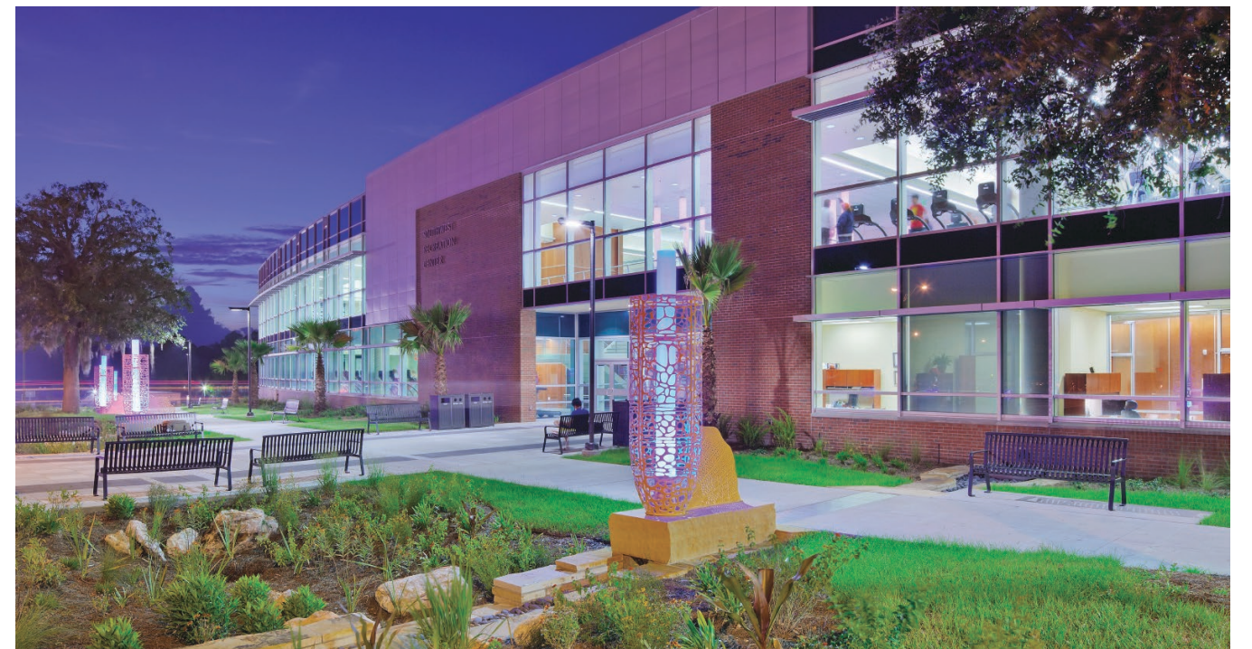
Figure 3.16 Steel Covered Runnels Spanning Sidewalk (IRIS22 Productions & RDG Planning & Design 2010). Used with permission
