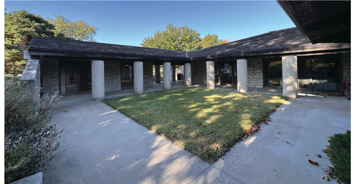
Figure 2.16 The Central Courtyard and Thick Concrete Pillars are a Primary Feature of the International Student Center (Tilley 2024).
