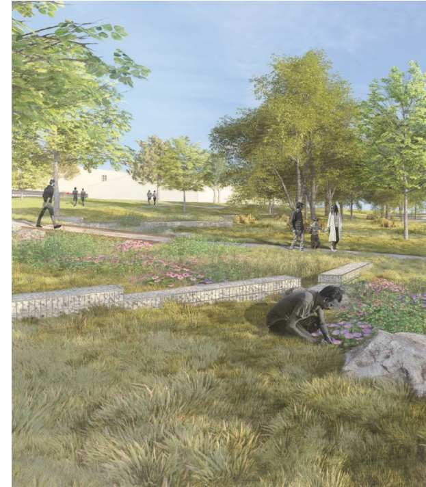
Figure 4.54 Gabion Check Dams help Slow Water (Freelove 2025).
