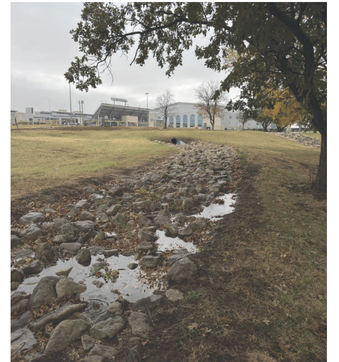
Figure 2.13 Rock Channels During Rain Event (Freelove 2024).
