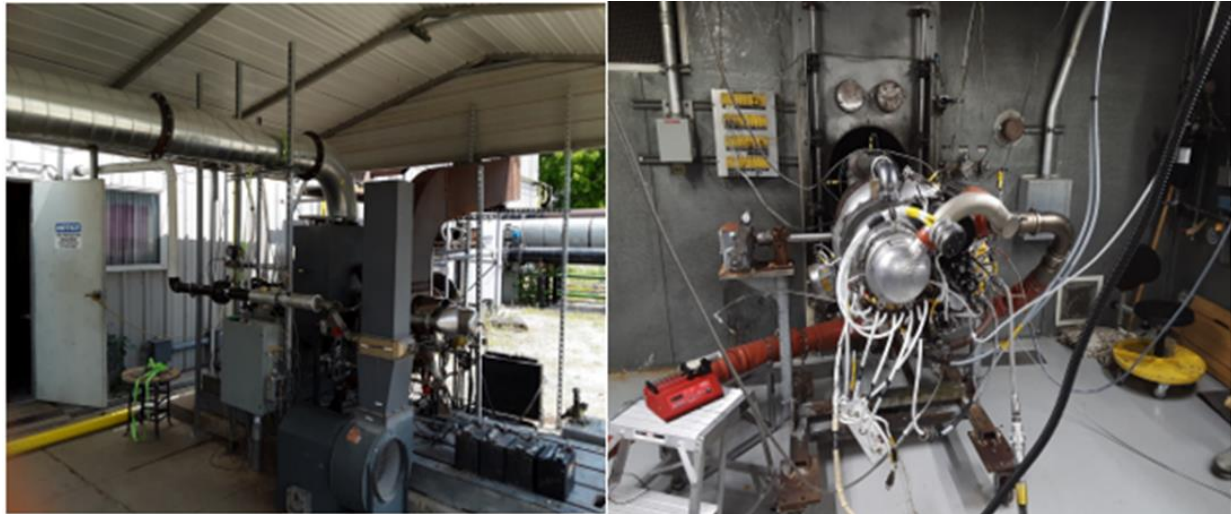
Figure 4-Allison 250 location/Testing Site and APU For ASHRAE 1830-RP
