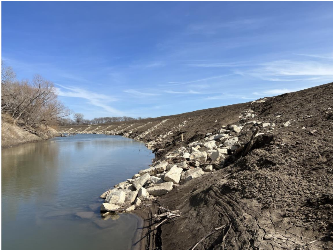
Figure 1.2 Downstream view of rock vanes on the Cottonwood River, Kansas.
