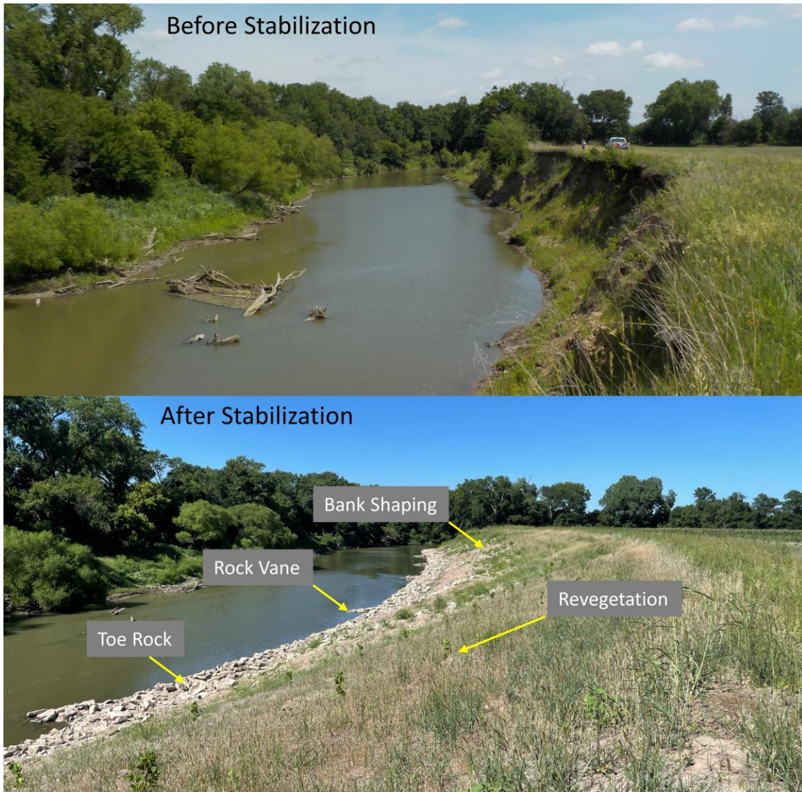
Figure 2.2 Downstream view of the before and after construction at C112 illustrating the SBS techniques used on both C112 and C102.
