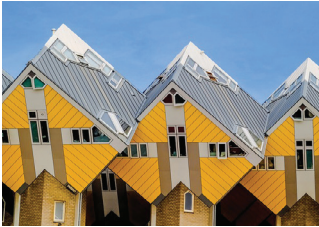
Figure 58: The iconic Cube Houses line one side of Oude Haven.
