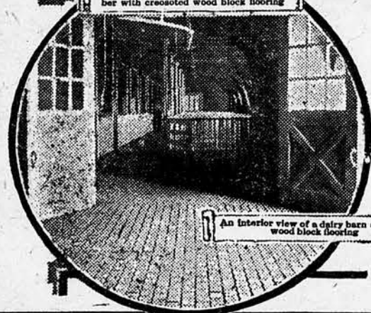
A cattle barn built of Southern Pine lumber with creosoted wood block flooring
