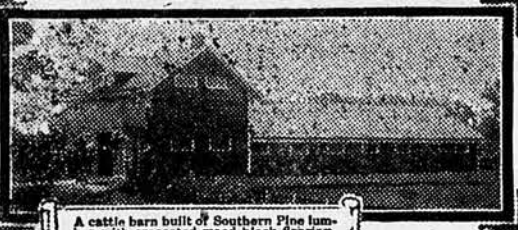
A cattle barn built of Southern Pine lumber with creosoted wood block flooring
