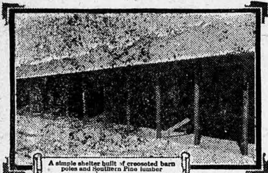
A simple shelter built of creosoted barn poles and Southern Pine lumber
